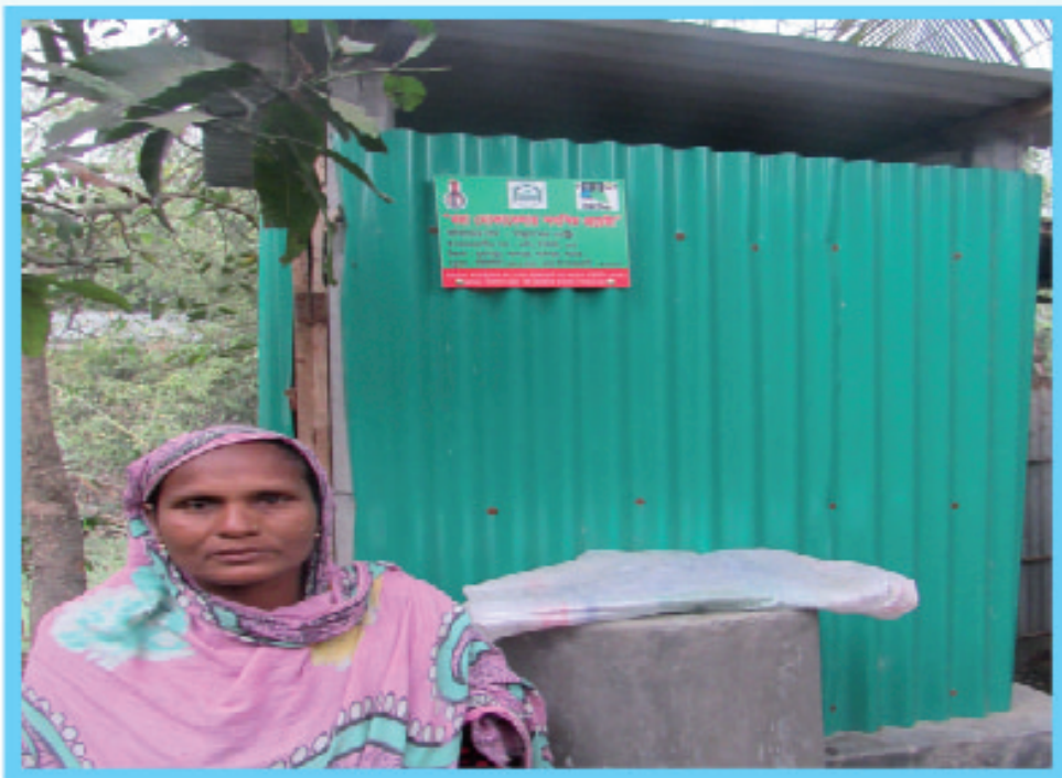
Photo 25: Mabia, in front of CCCP installed sanitary latrine
